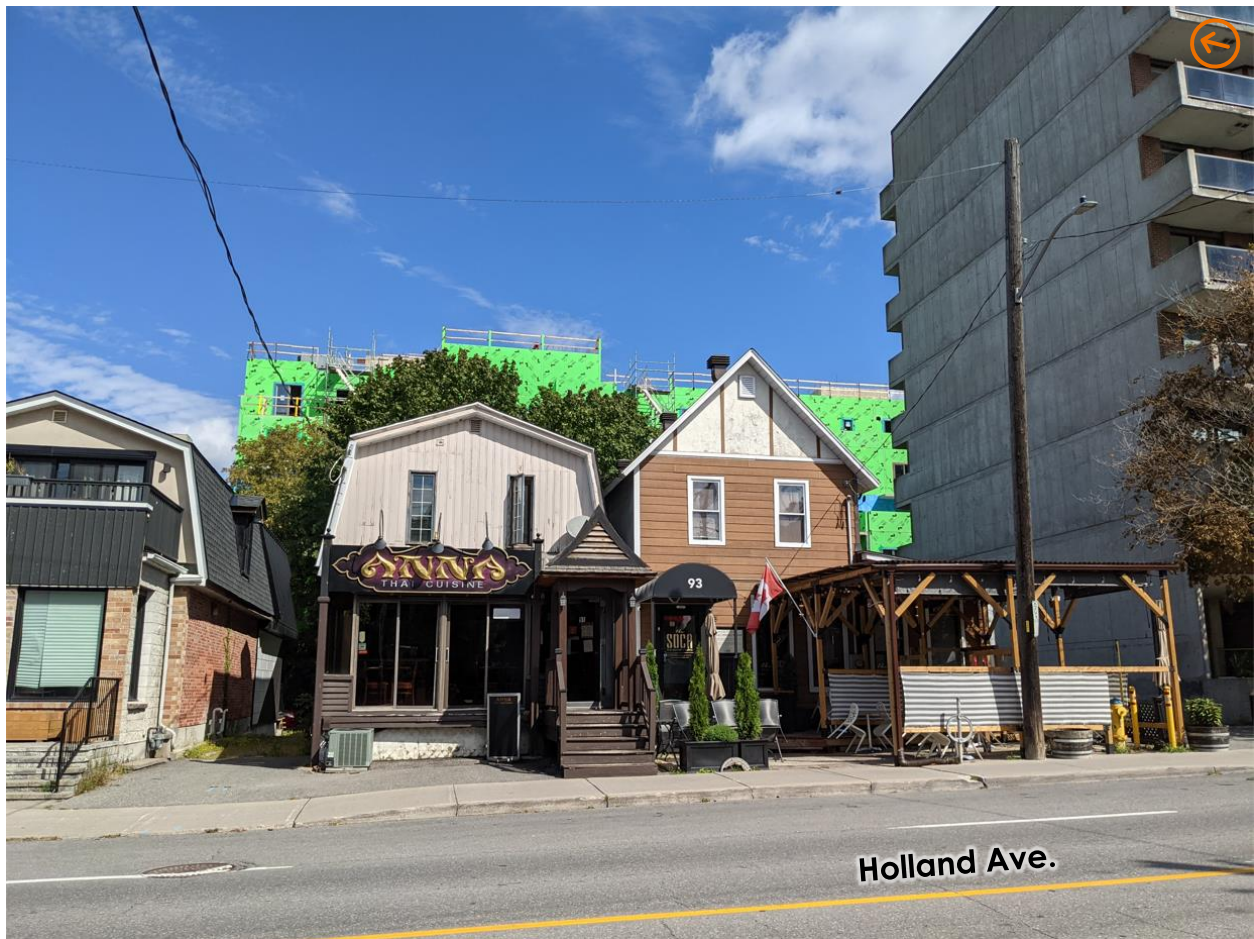
FIGURE 6. STREETVIEW OF THE SITE FACING EAST (SEPTEMBER, 2021)
