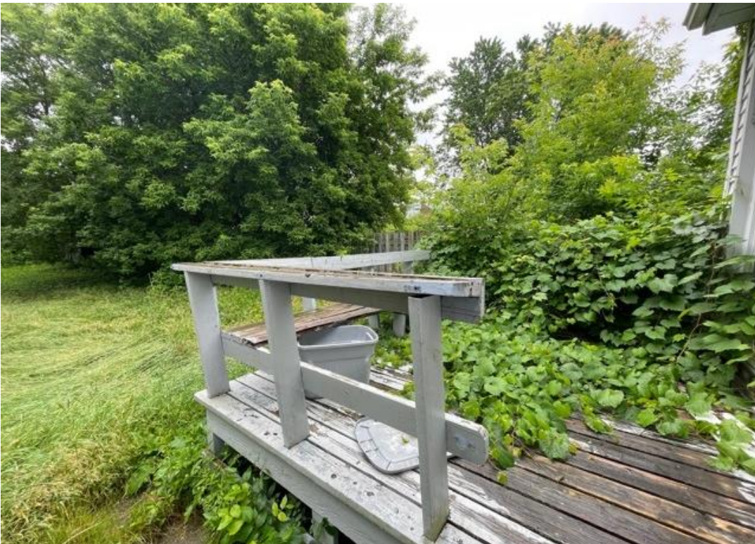
Photograph 2: View of the east side of the dwelling, looking southeast.
