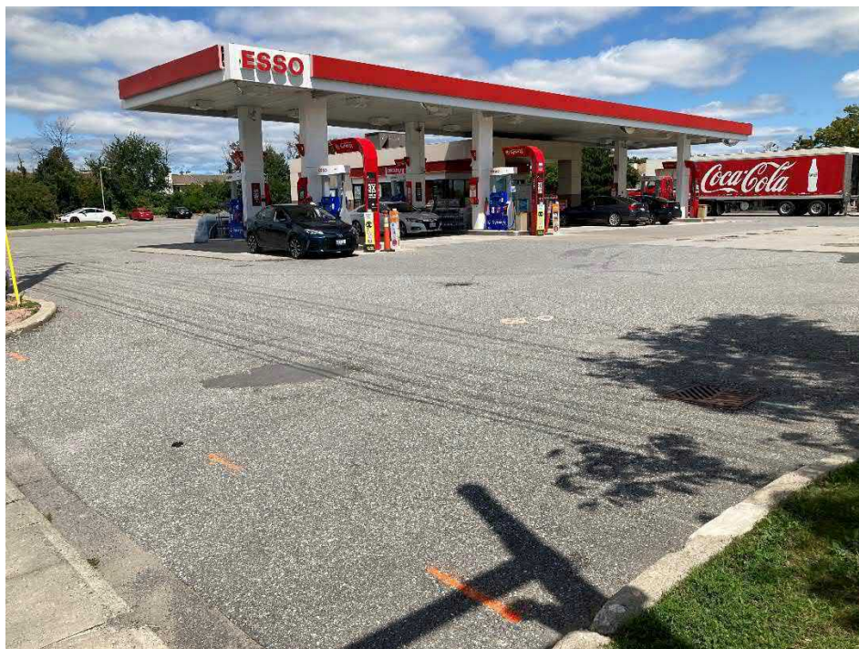
Photo 2: View of the fuel pumps, canopy, tank nest (background) and on-site catch basin (foreground)
