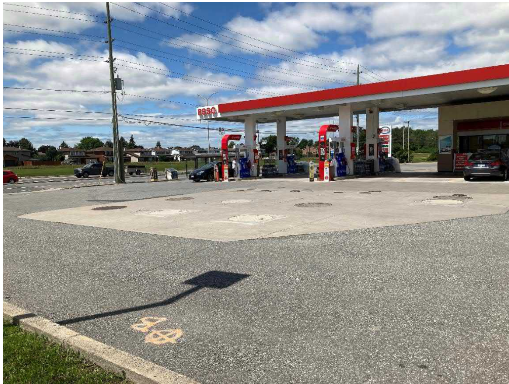
Photo 5: View of the tank nest (foreground), fuel pumps and Woodroffe Avenue (background)
