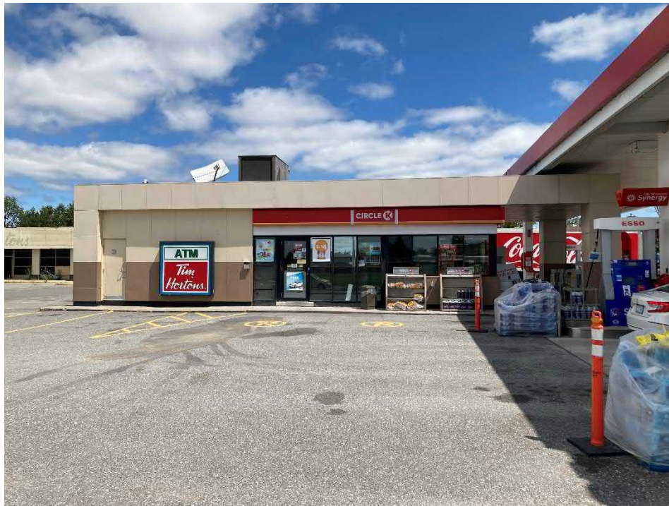
Photo 1: View of the west-facing retail fuel outlet and fuel pumps (left)
