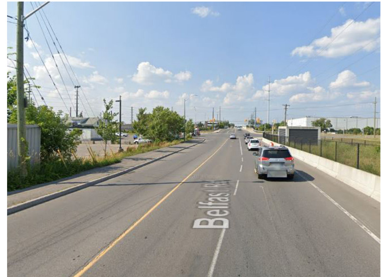
4. Looking North on Belfast South of Tremblay
