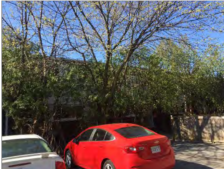
Photo 1 – Site Building (north elevation).
