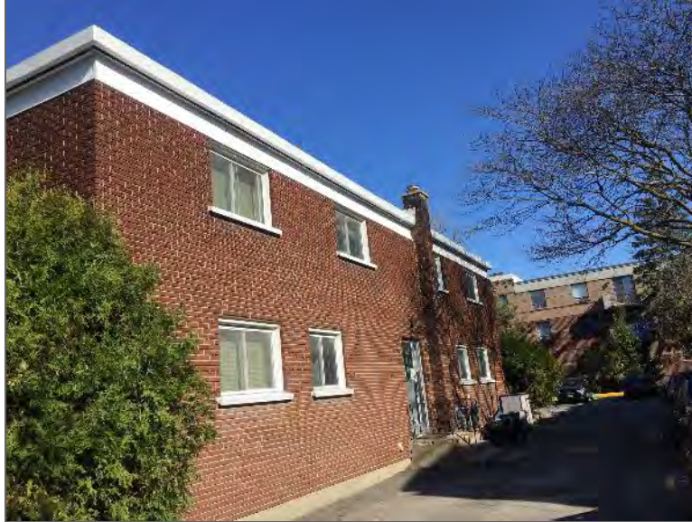
Photo 3 – Site Building (east elevation).
