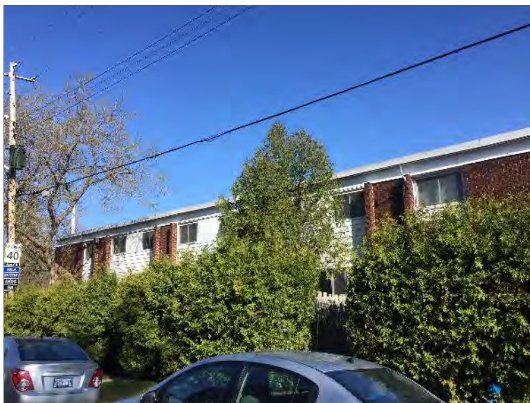
Photo 2 – Site Building (south elevation).
