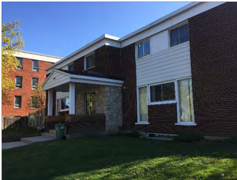
Photo 4 – Site Building (west elevation).
