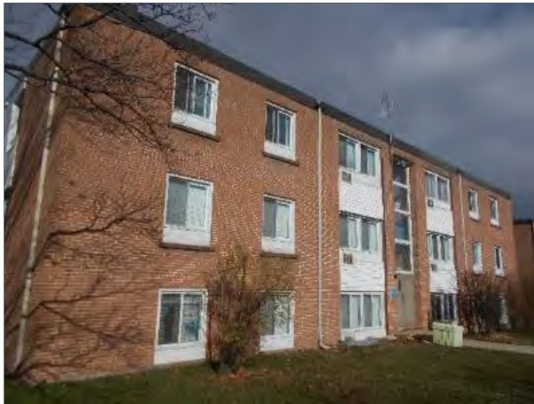
Photo 2 – Site Building B (south elevation).
