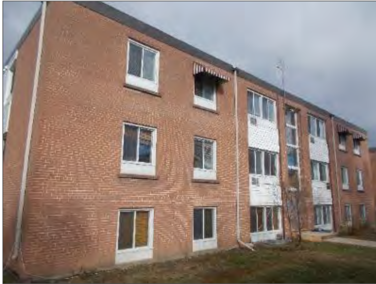
Photo 1 – Site Building A (south elevation).
