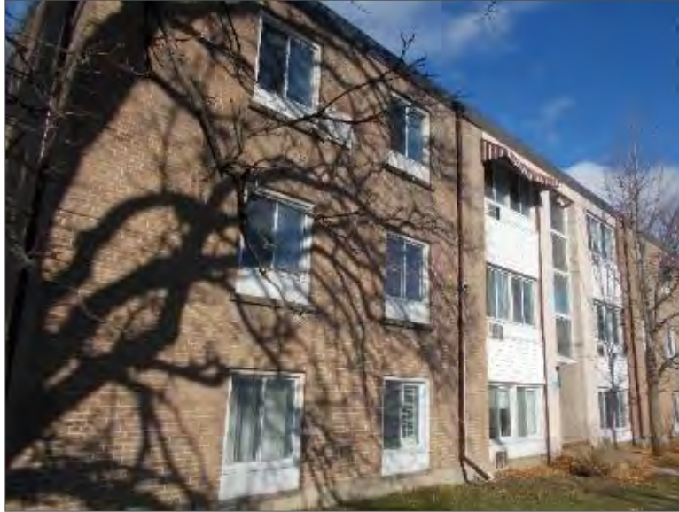
Photo 3 – Site Building C (south elevation).
