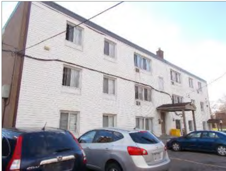
Photo 4 – Site Building C (north elevation).
