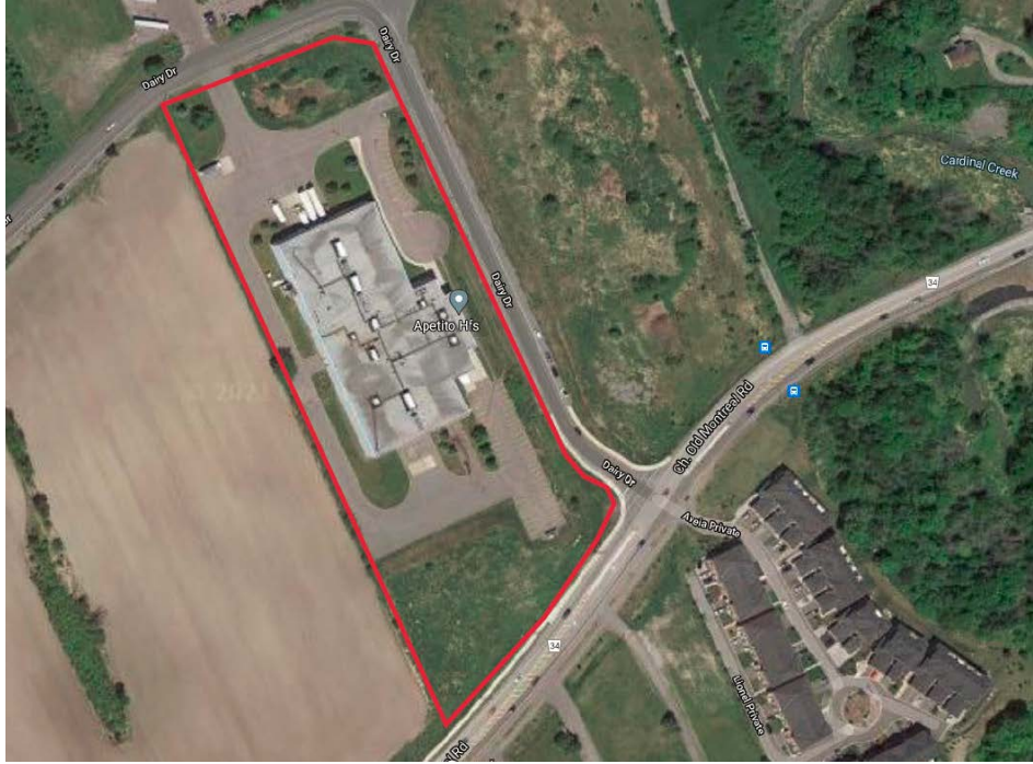
Figure 1: The Subject Property with Lot Lines Approximated in Red
