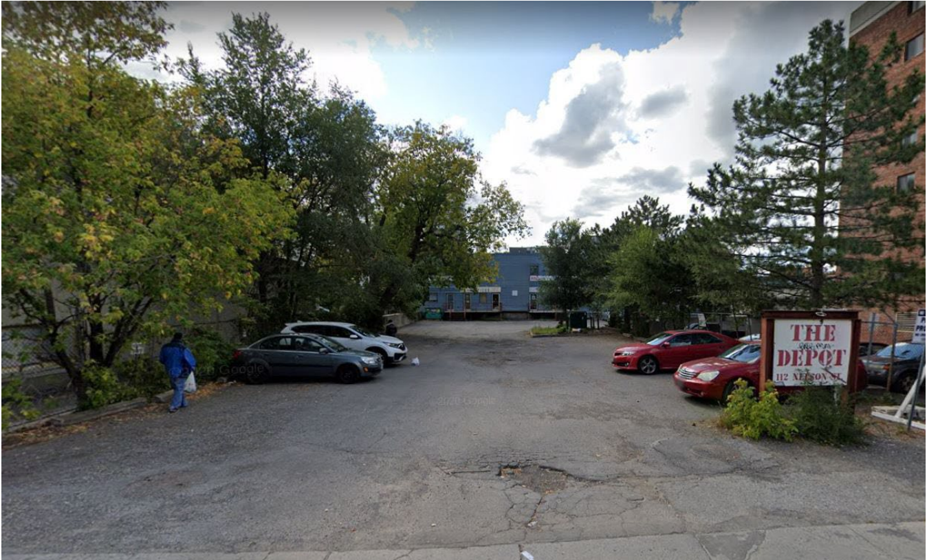
Figure 2: Existing three-storey mixed use building on the subject property
