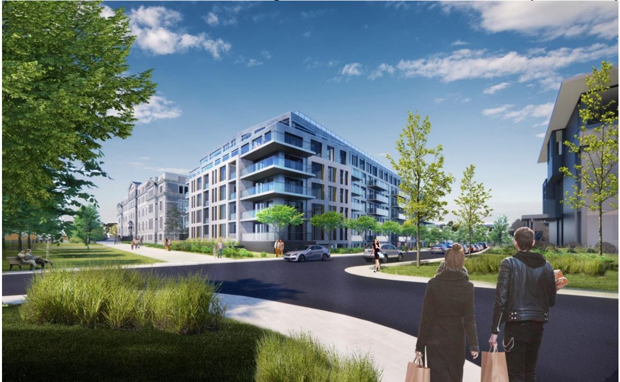
Figure 16. View from Deschatelets Avenue (south facade)
