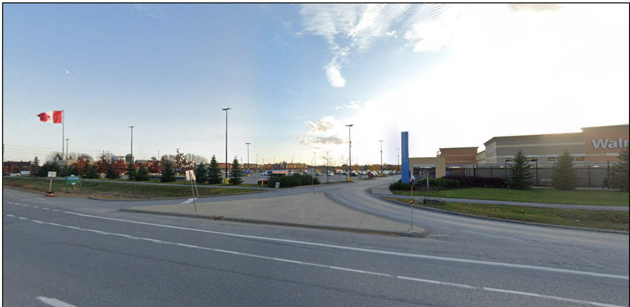
Figure 4: The Shopping Plaza west of the Subject Site, across Terry Fox Drive.
