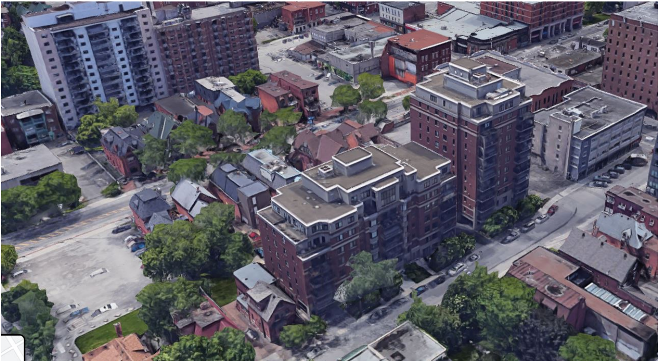
Figure 14 Newer 7 and 11-storey buildings with frontage along Cooper Street.
