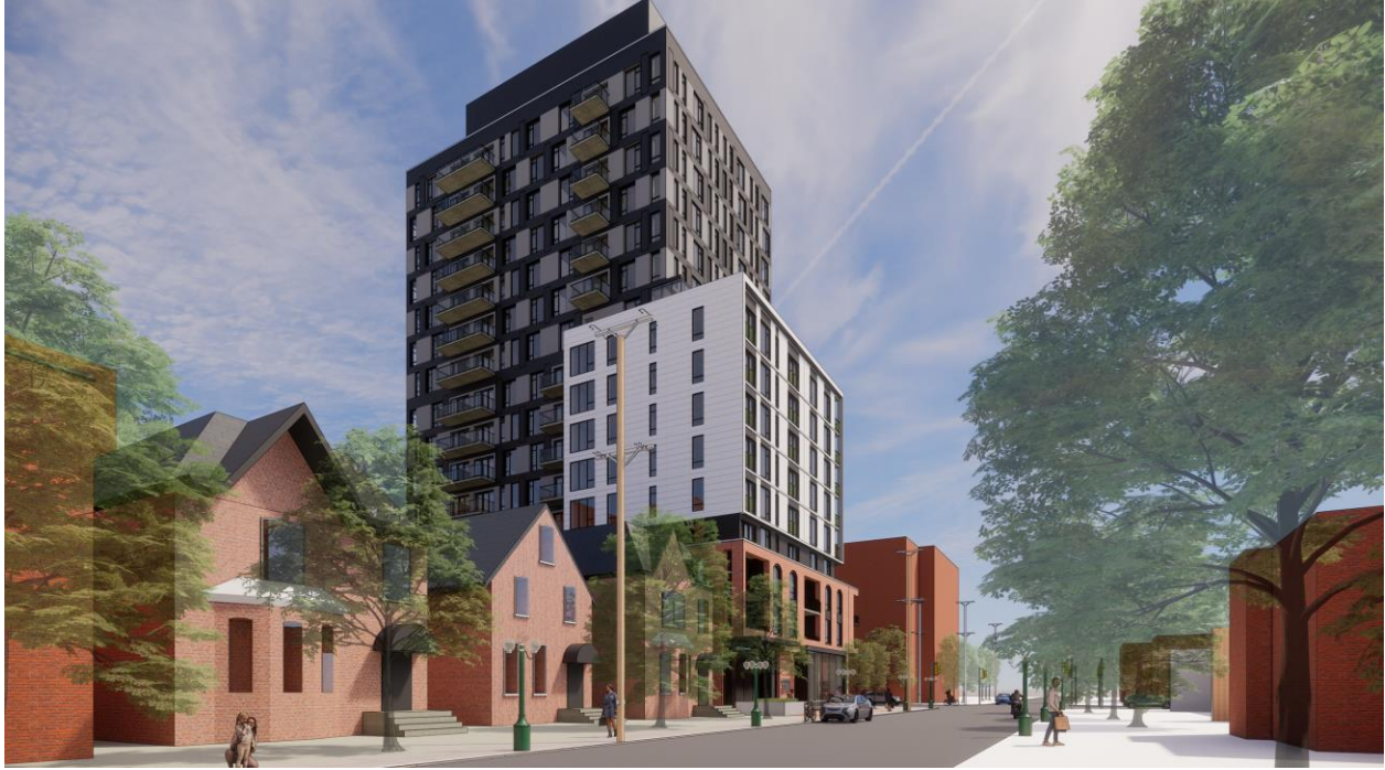
Figure 14: View looking north east of the proposed development illustrates the stepping of the tower and the integration of the development along Somerset with the defined step backs and material changes.
