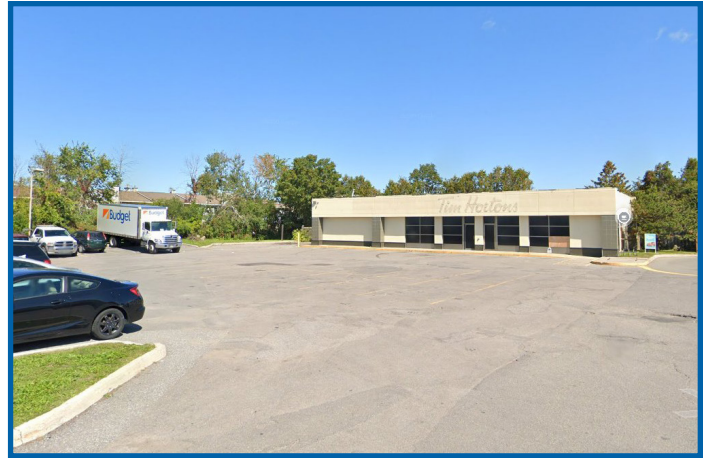
Figure 2.0d - Existing vacated one storey retail building (Tim Hortons)
