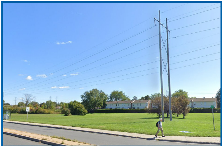
Figure 2.0j - Hydro corridor on south side of Medhurst Drive
