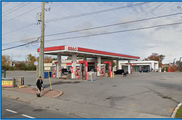
Figure 2.0c - Existing 1 storey gas bar on site
