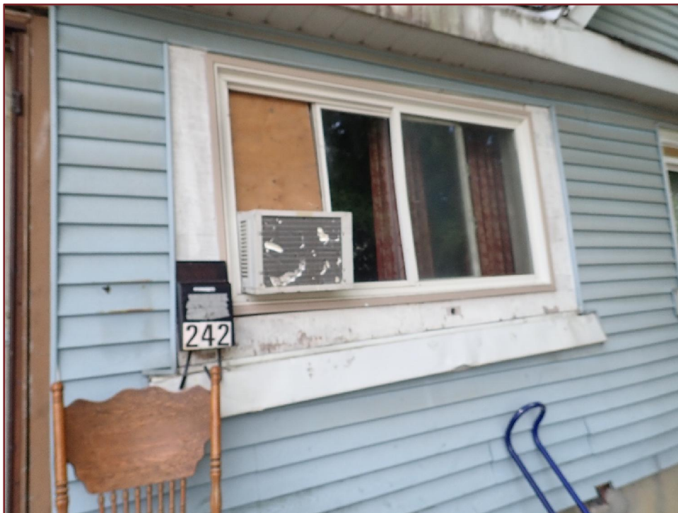
Photograph 6 Representative photograph of window air conditioners located within the subject property building
