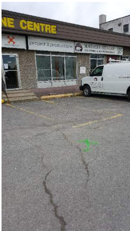
2.2 BH2017 – 2 location, looking North.
