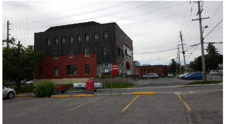
1.2 BH2017-1 Location looking direction South
