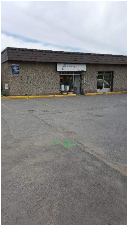
1.1 BH2017-1 Location looking direction North.
