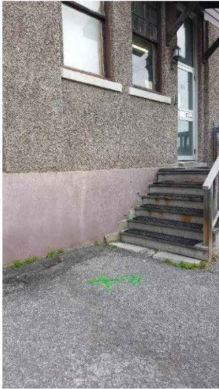
3.1 BH2017-3 Location looking North East.
