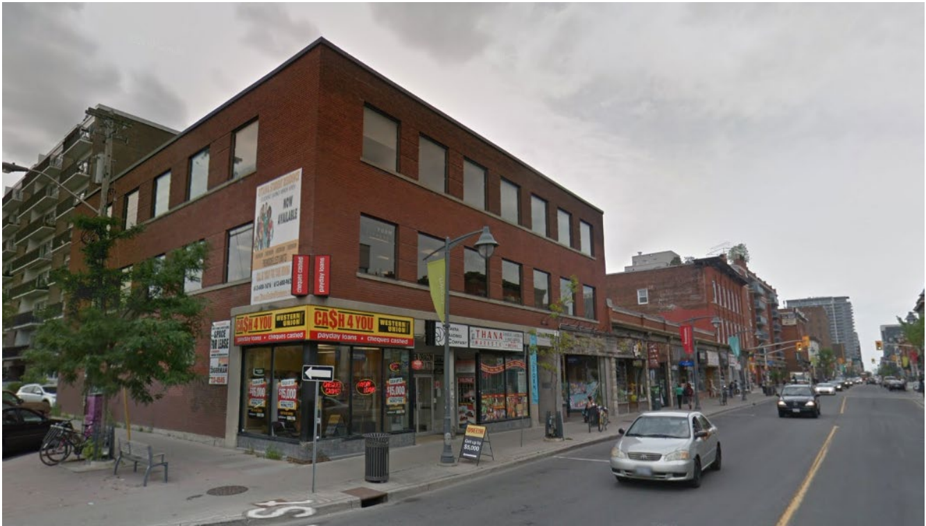
Figure 9: Property at 382-386 Bank Street, north of the subject site, showing materiality, window openings, and scale similar to the proposed design
