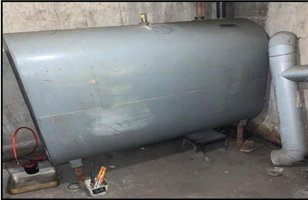
Photograph 3: View of an aboveground furnace oil storage tank, located in the basement of the subject building.
