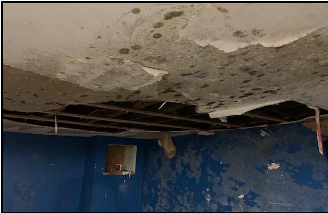
Photograph 4: View of water damage and mould growth, located in the basement of the subject building.
