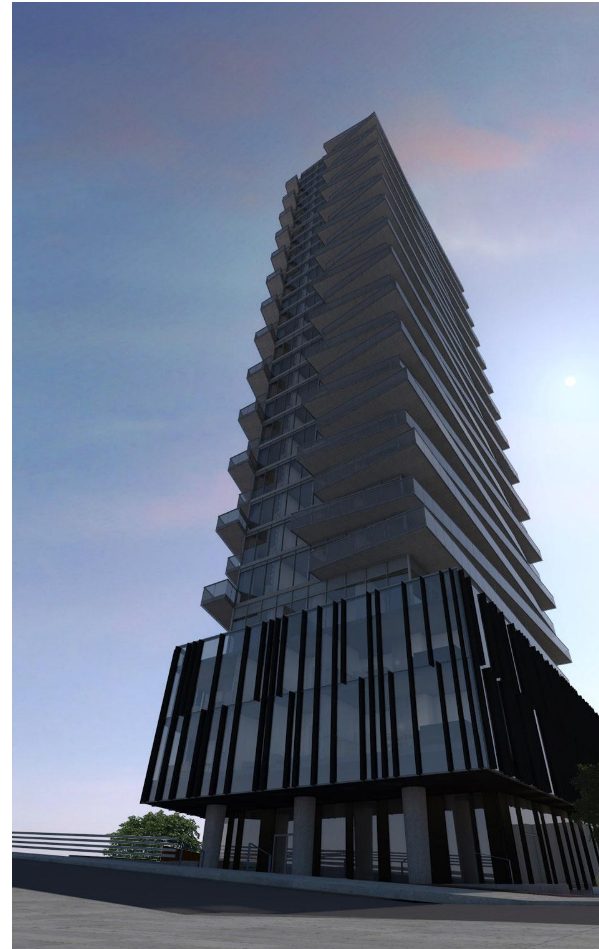
North West Corner
