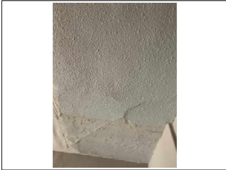
Photograph 7: View of suspected asbestos-containing stipple ceilings throughout the subject building.
