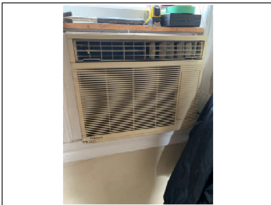
Photograph 10: View of window air conditioning unit on the second floor, suspected to contain ODSs.
