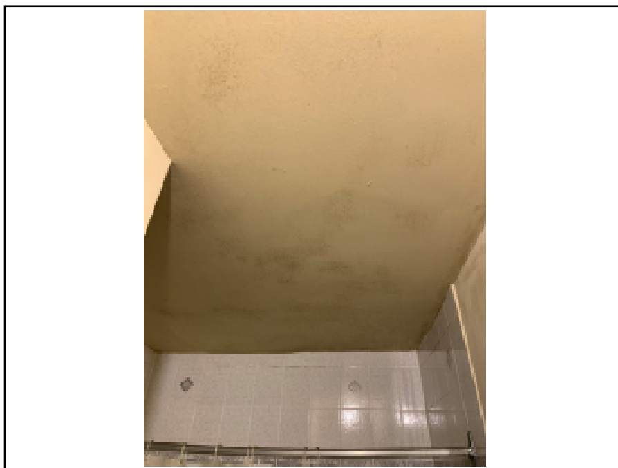
Photograph 11: View of visible mould in the main floor washroom.
