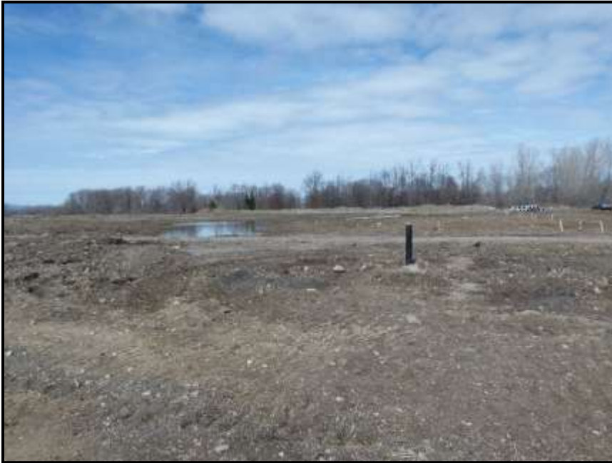
Photograph 1: Looking north across Block 1 (April 4 th , 2020).
