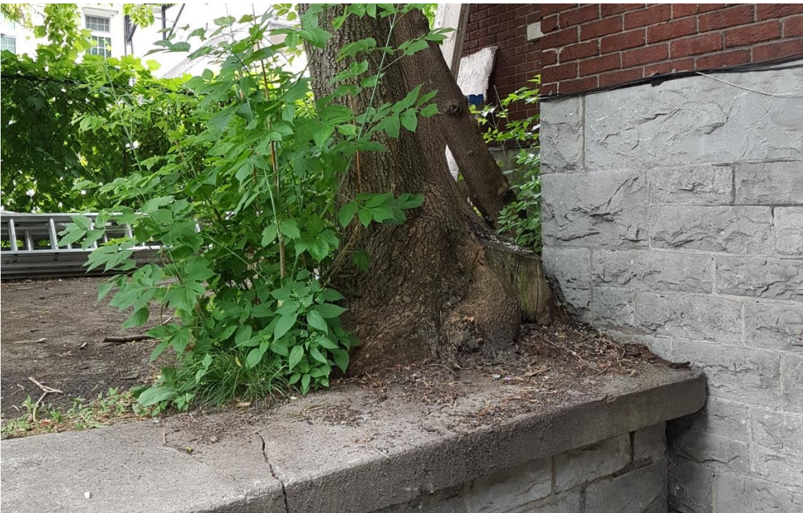
Photo C: Showing root system of a Manitoba Maple undermining the foundation of the existing building as well as the existing retaining wall.
