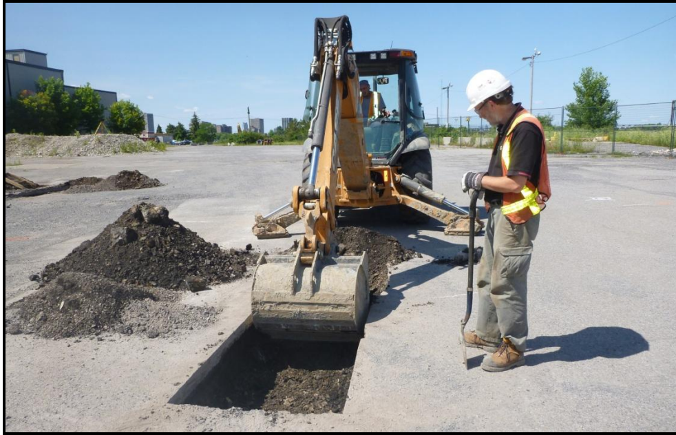
Image 3. Staff monitoring the mechanical excavation of Trench 1C, facing west. (PR15-24D019)
