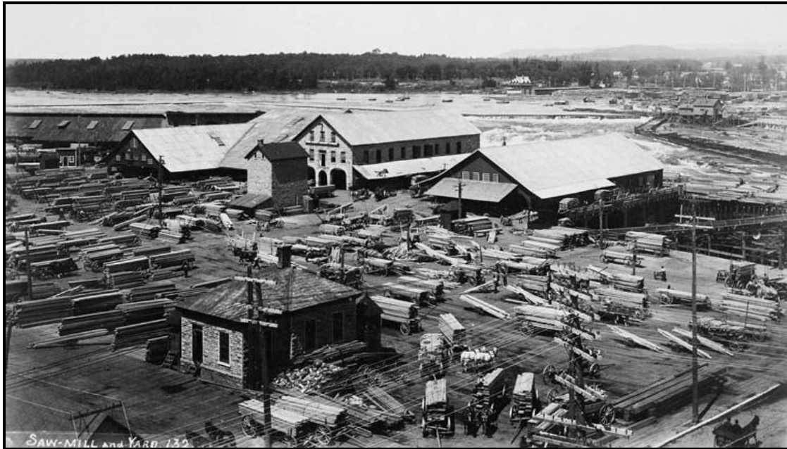
Image 24. The J.R. Booth sawmills and yard at the Chaudière Falls c. 1900, facing northwest. (LAC C-003017) The building in the foreground is the J.R. Booth office, which survived the Great Fire. To the rear of this is the hose house. The hole in the ground (rear right) is where the concrete hydro-electric power station now stands.
