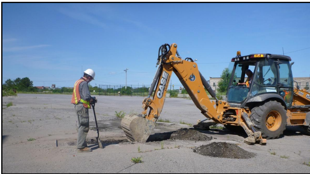
Image 2. Staff monitoring the mechanical excavation of Trench 1A, facing northwest. (PR15-24D013)
