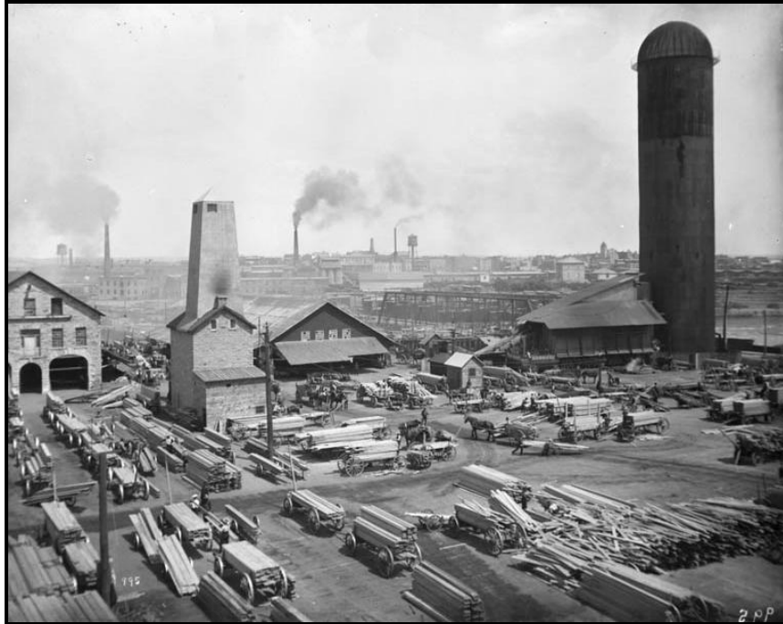
Image 26. The J.R. Booth lumber mill and yard on Chaudière Island in 1907, facing northeast from the new boiler house. (LAC PA-008960) The newly erected, brick-lined waste burner is on the right. The study area is partially shown in the bottom right of the photograph.
