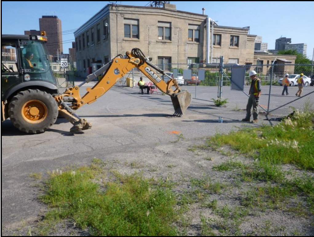
Image 1. Staff monitoring the mechanical excavation of Trench 1E, facing northeast. (PR15-24D002)
