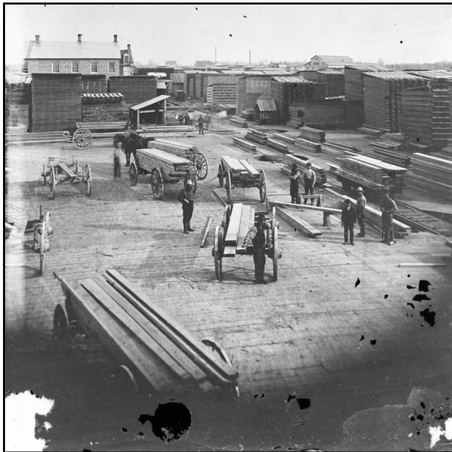
Image 23. The Perley and Pattee lumber yard on Chaudière Island in 1878. (LAC PA-012571) This early photograph best illustrates the convention of covering the ground with wooden planks within the lumber yard to facilitate the transport of lumber around the site. Horse tram lies are also visible on the right running north-south and in the distance running east-west.
