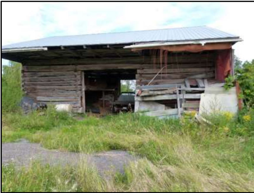
Photograph 27: Building #8 – no Barn Swallow nests were noted (August 14 th , 2017).
