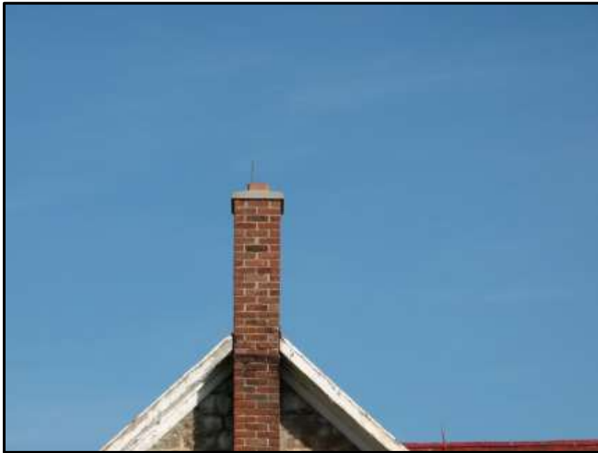
Photograph 29: 910 March Road (Building #1) chimney with ceramic liner (August 14 th , 2017).
