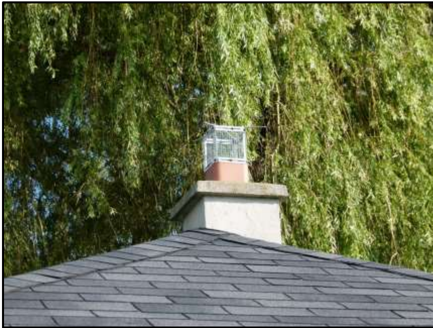
Photograph 31: 920 March Road (Building #5) chimney with metal cap (August 14 th , 2017).
