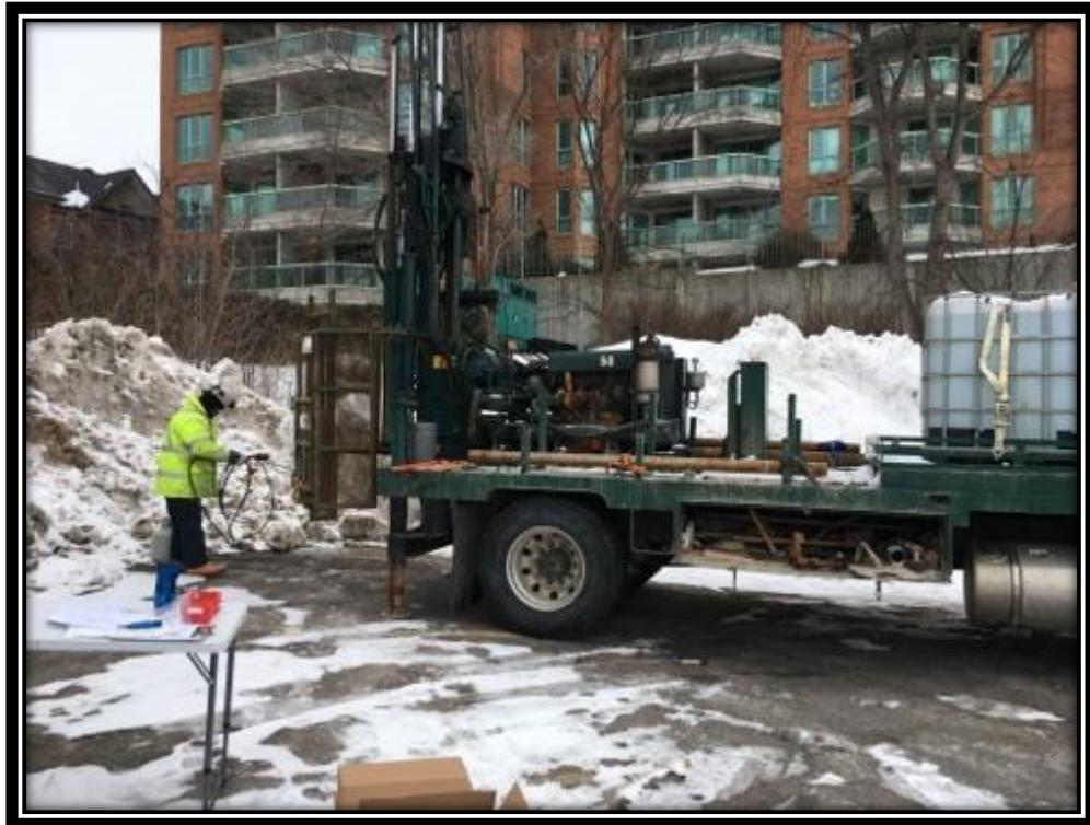
**Photograph 2:** View of drilling activities at MW17-01, facing northeast (Feb 11, 2017)
