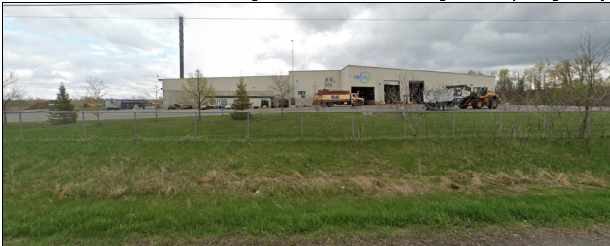
Figure 3. Renewi Canada Ltd. Organics Composting Facility
