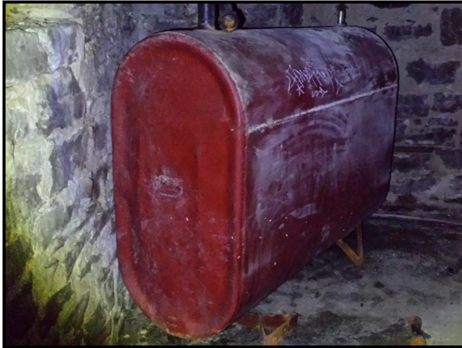
Photograph 5: View of an empty oil tank, located in the basement of the abandoned farmhouse on 4055 Russell Road.
