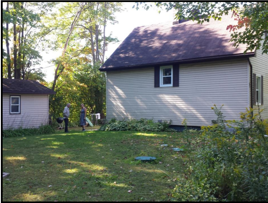
Photograph 7: View of the private septic tank cap, located on the exterior the occupied residence situated on 4055 Russell Road (addressed 3995 Russell Road).
