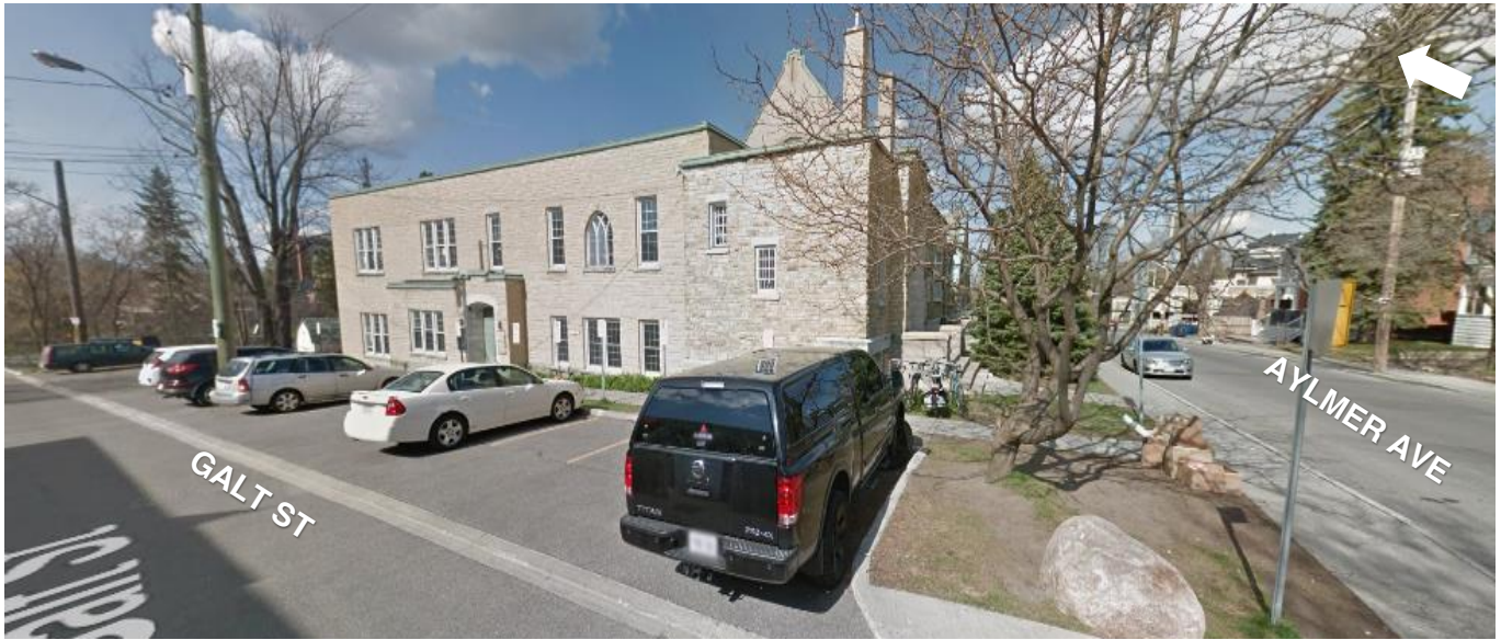
Image 13. Facing northeast from the intersection of Galt Street and Aylmer Avenue
