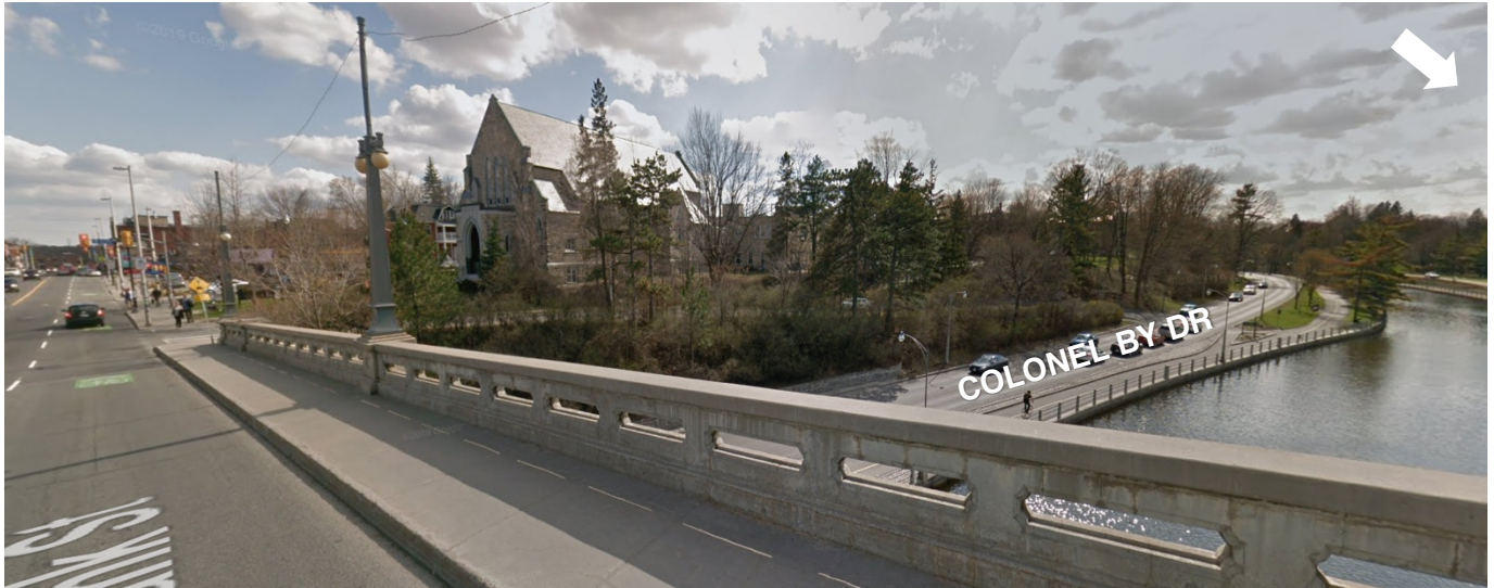
Image 1. Facing southwest towards the church from the Bank Street bridge
