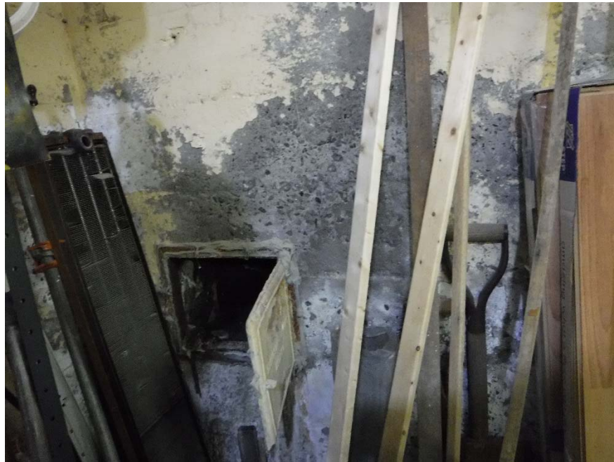
Photo 15. Chute observed in the old boiler room, located below the basement of the west church building.
