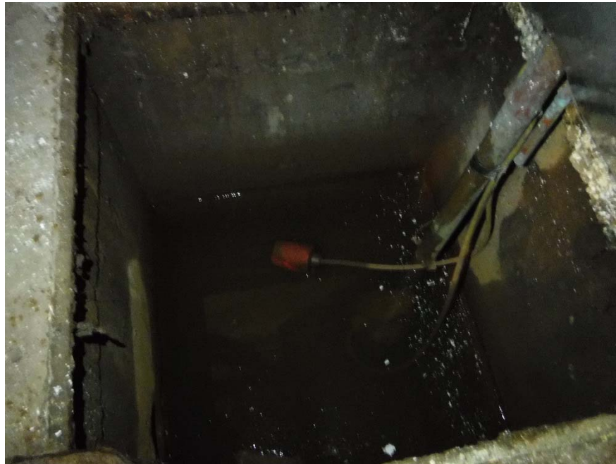
Photo 13. Water in sump pit, located in the boiler room.
