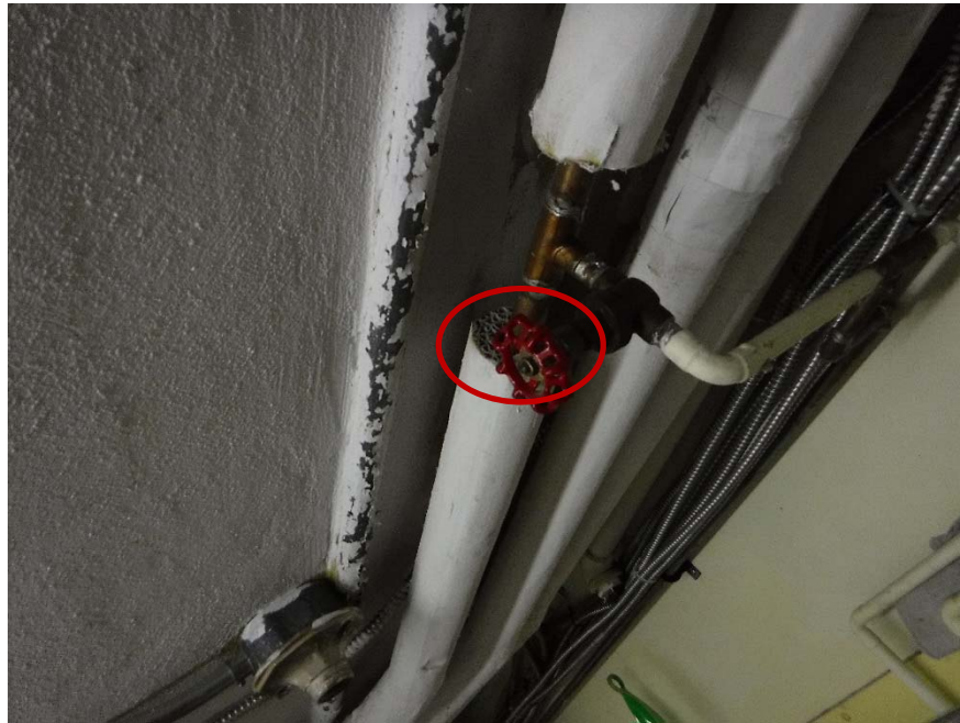
Photo 11. Pipe wrap suspected to contain asbestos and ceiling texture coat, located in the boiler room.
