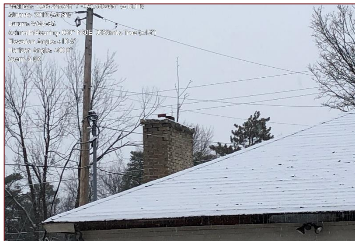
Site Photograph 7 – Capped Chimney
