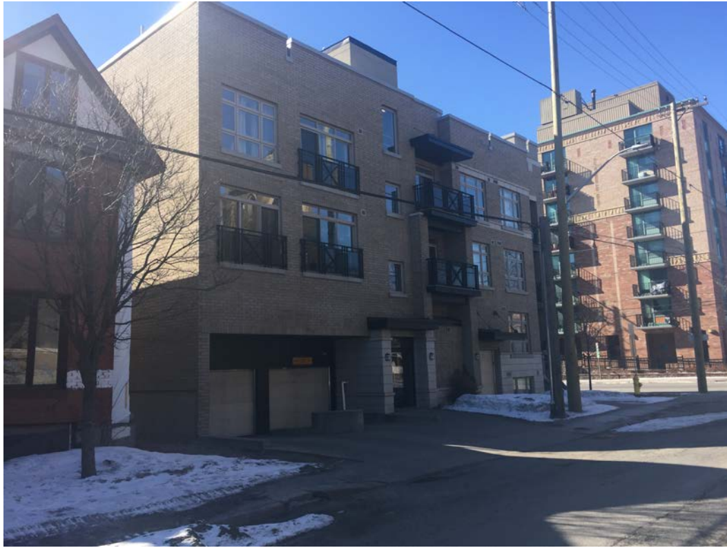
Existing Residential building located immediately west of site
