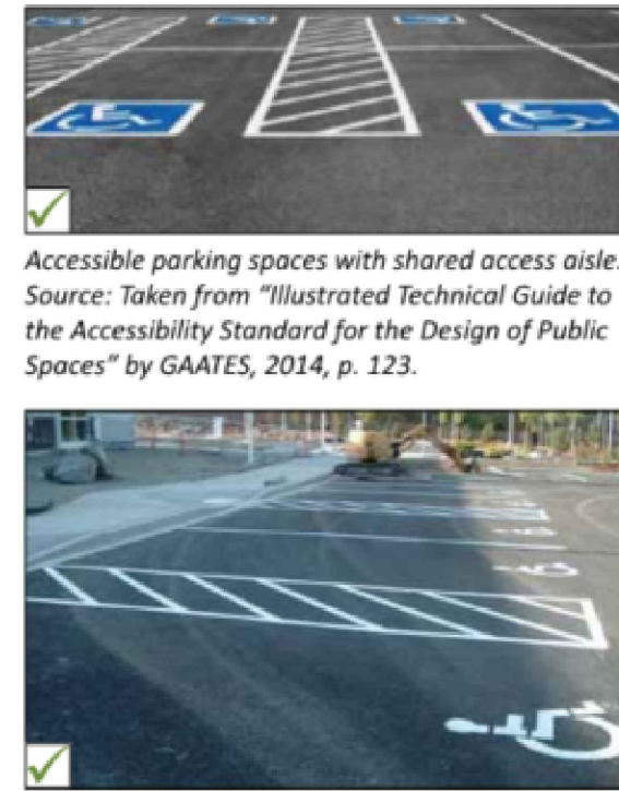
Accessible parking spaces with shared access aisle and curb ramp. Source: Taken from "Illustrated Technical Guide to the Accessibility Standard for the Design of Public Spaces" by GAATES, 2014, p. 123. Accessible parking spaces with access aisle and curb ramp. Source: Taken from "Illustrated Technical Guide to the Accessibility Standard for the Design of Public Spaces" by GAATES, 2014, p. 115.
