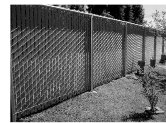
7 1.8m Chain Link Fence w/ Vinyl Slats DP1.02 SCALE: NTS
