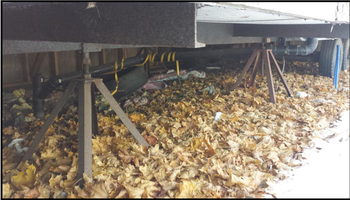
Photograph 5: View of a septic drainage pipe located underneath the portable office trailer.
