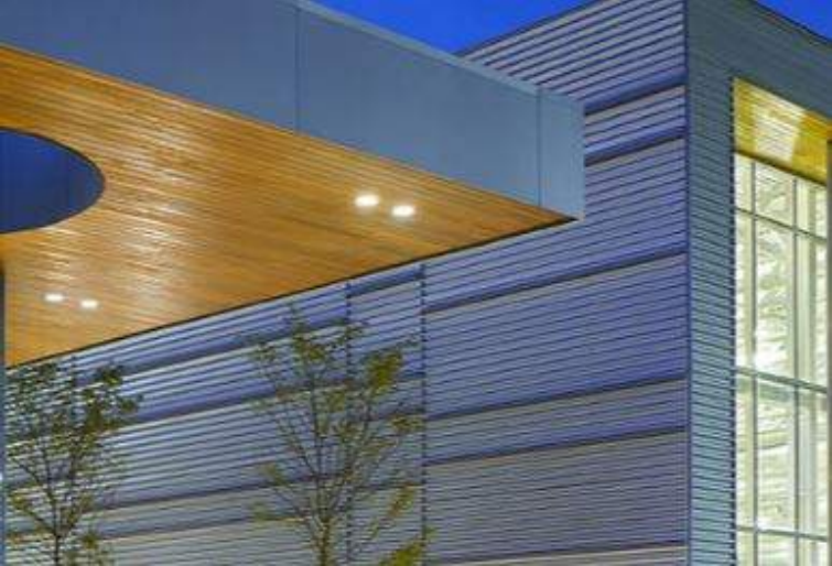
Wood Look (Metal) Soffit Colour: Oak 7/8" Corrugated Steel Panels Colour: Grey / Silver
