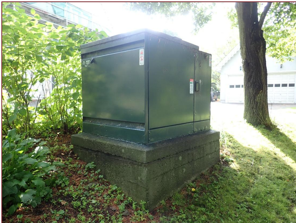
Photograph 14 Green concrete pad mounted transformer located on side
