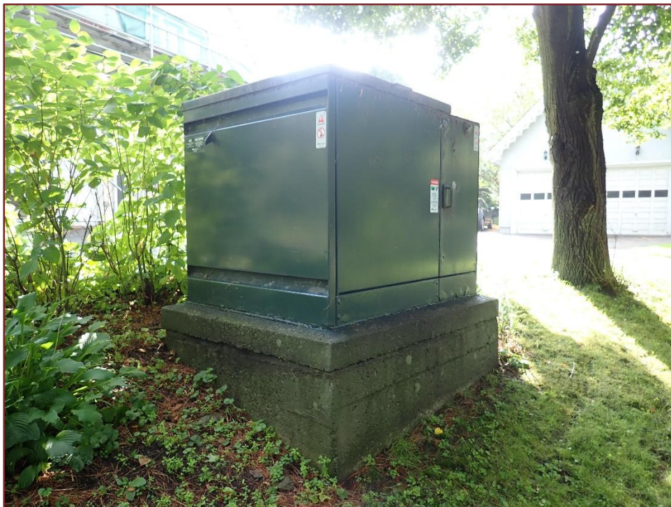
Photograph 16 Green concrete pad mounted transformer located on side
