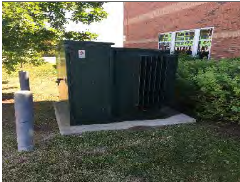
Photo 6 – Pad-mounted oil-cooled transformer located on the northwest portion of the Phase One Property (PCA #1).
