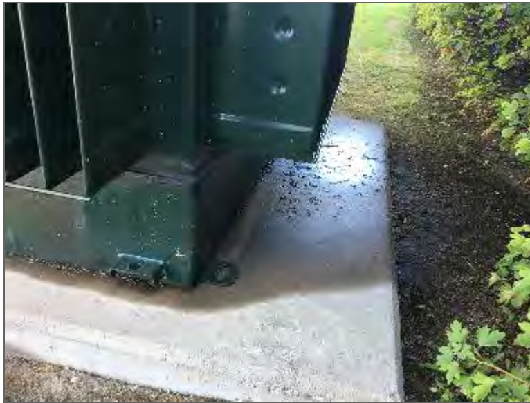
Photo 7 – Dark staining observed in the vicinity of the above-noted pad-mounted oil-cooled transformer depicted in Photo 6. It should be noted that this was addressed as part of the 2019 Hemmera Remedial Excavation Report.
