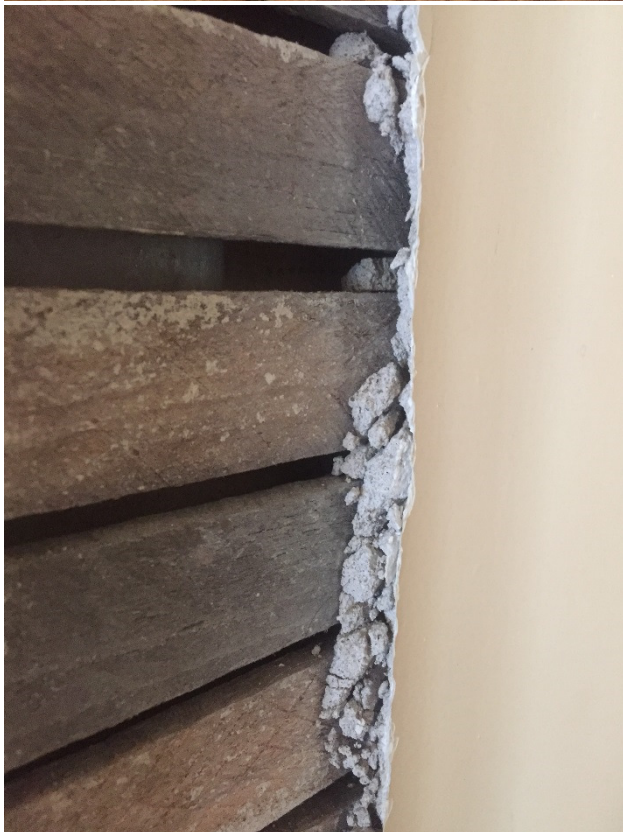
Photo 4 – Plaster walls in a poor state of repair.
