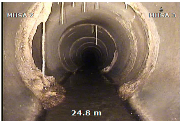
Figure 14 – Encrustation at pipe joints
