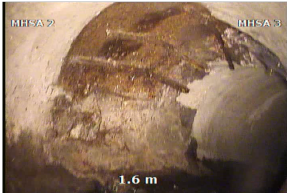
Figure 12 – Rebar exposed at MH-pipe joint
