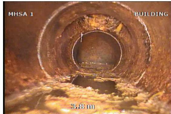
Figure 5 – Sanitary backflow in abandoned storm service
