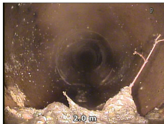
Figure 7 – Partial blockage (2.0m from MHSA1)
