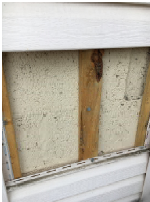
Photograph 24: View of painted concrete block behind siding on single storey section of building.
