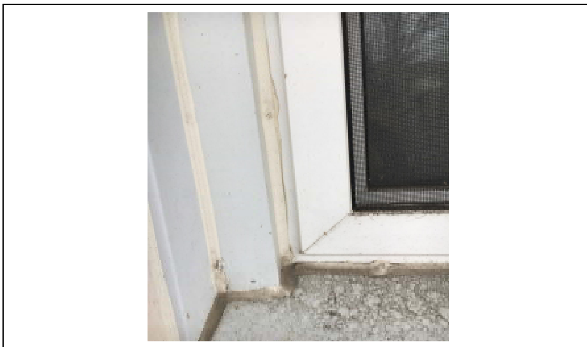
Photograph 25: View of outside caulking around windows of building.
