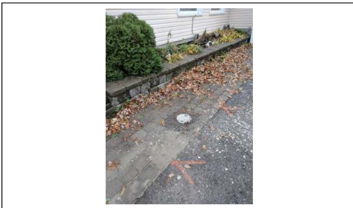
Photograph 26: View flush mount manhole cover protecting monitoring well on north side of building.
