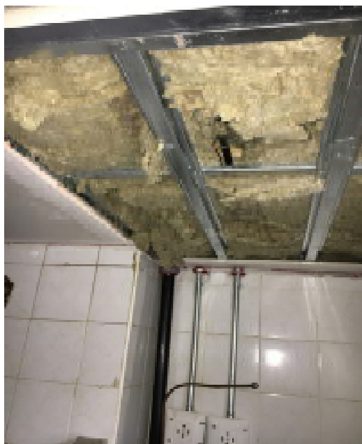
Photograph 15: View of insulation between kitchen ceiling and upstairs floor.
