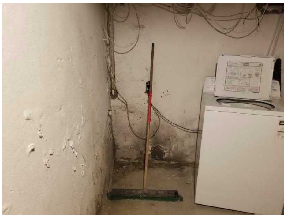
Photo 6: Potential mould-like substance found in the basement, beside the washing machine at 114 Russell Avenue.
