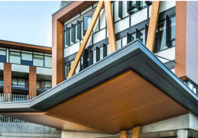
EW-4: “Longboard”, wood-look Aluminum soffit and window accent
