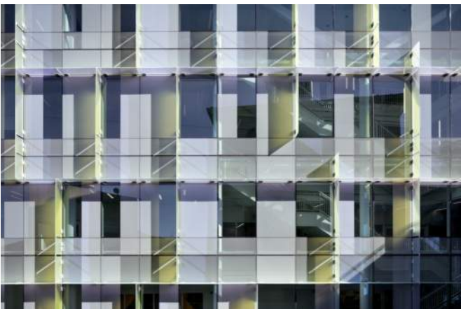
Silk-screened glazing frit for glare / heat gain reduction (40%, 50%, and 70% transmittance)
