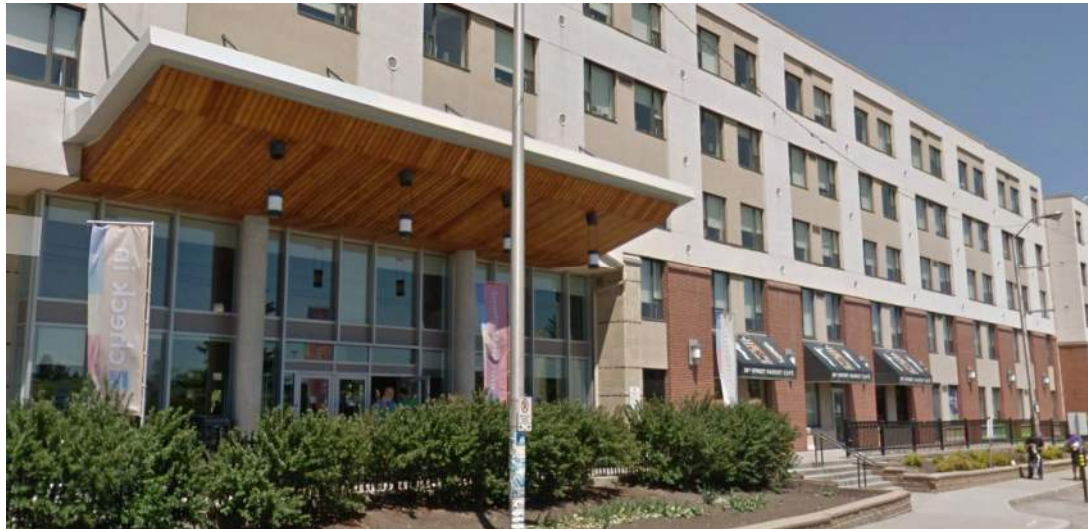
Wood Soffit and masonry / EIFS at Student Residence
