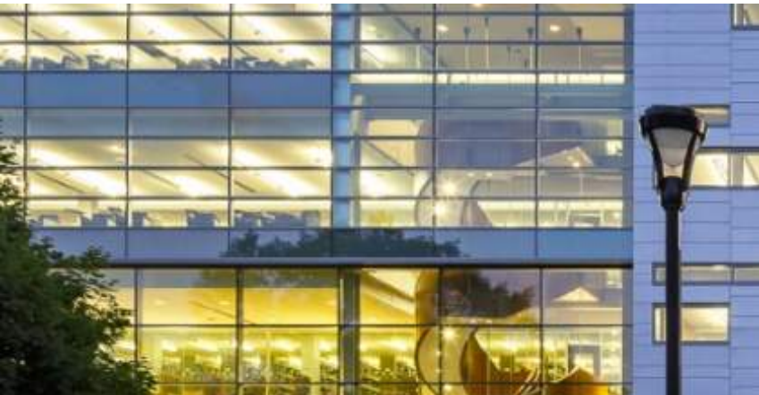
GL-1: Vertical silicone joint, horizontal black mullions
