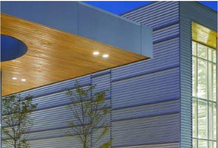
EW-3: 7/8” Corrugated Steel Panels Colour: Grey / Silver
