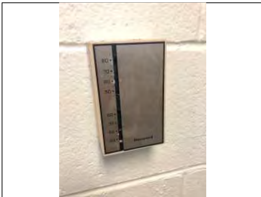
Photograph 20: View of thermostat containing mercury
