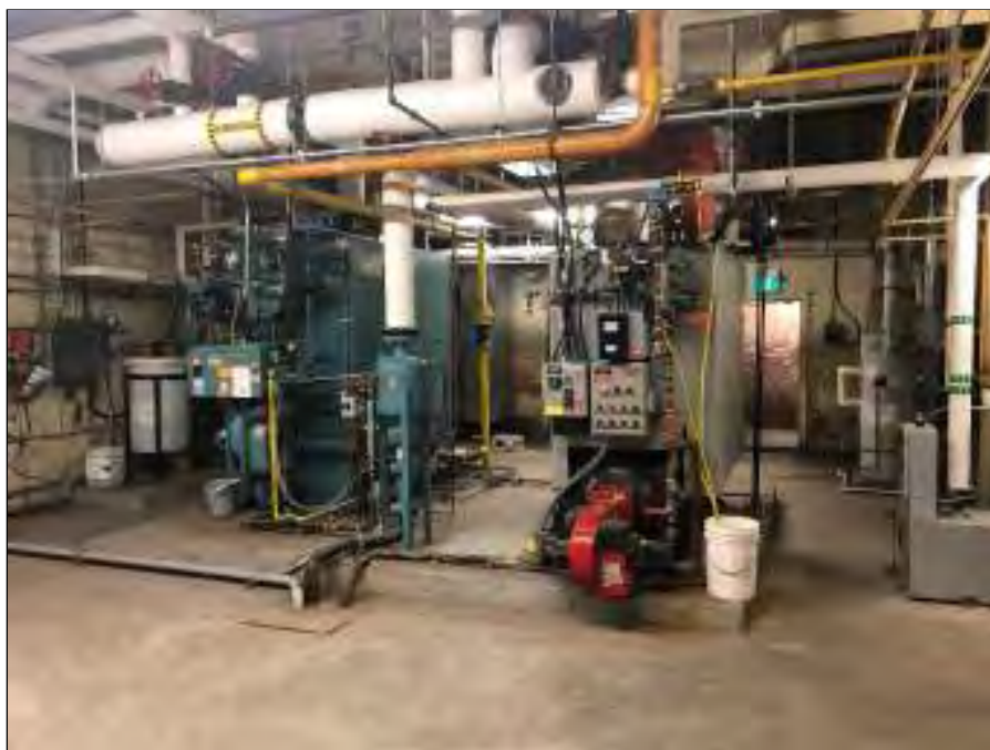
Photograph 16: : View of natural gas fired boilers
