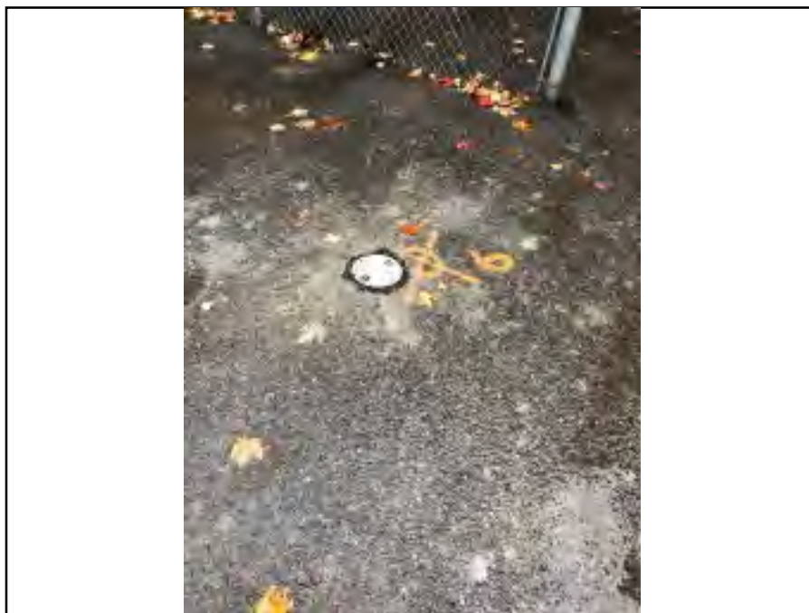
Photograph 11: View of exterior geotechnical monitoring well
