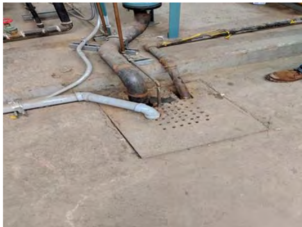
Boiler Drain
