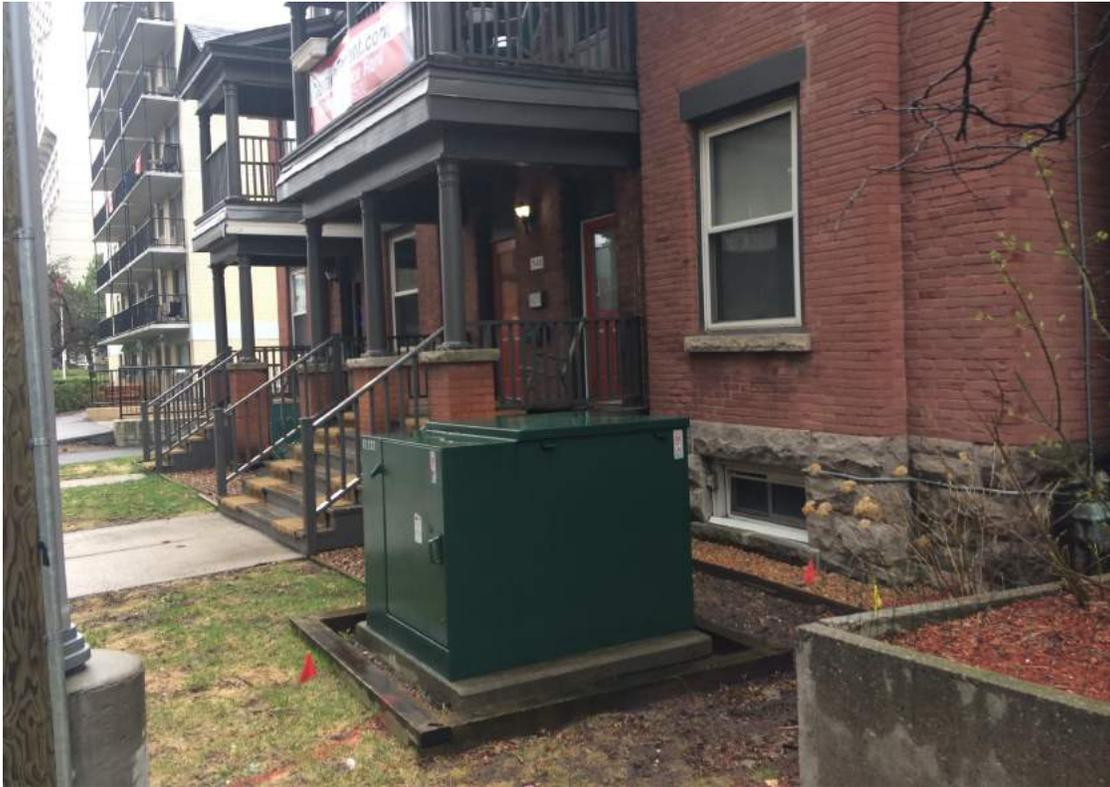
Photograph 3: Transformer and natural gas connection at the southeast corner of the subject structure.
