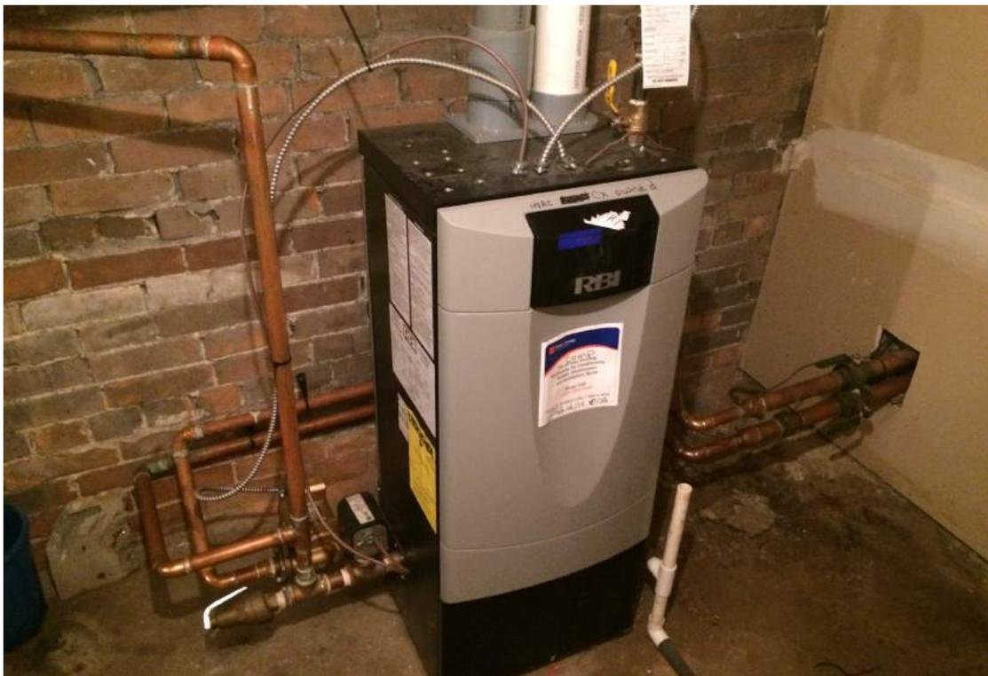
Photograph 4: Natural gas boiler located in the basement of the subject building.
