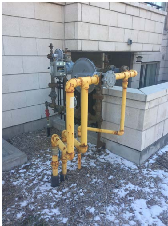
View of natural gas meters for residential building located immediately west of 32 Florence Street
