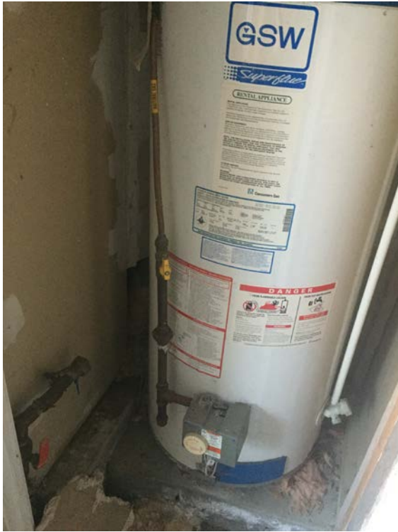
View of disconnected natural gas water heater in basement
