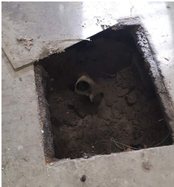
Photograph 6: View of the garage bay floor pit with drainage pipe.
