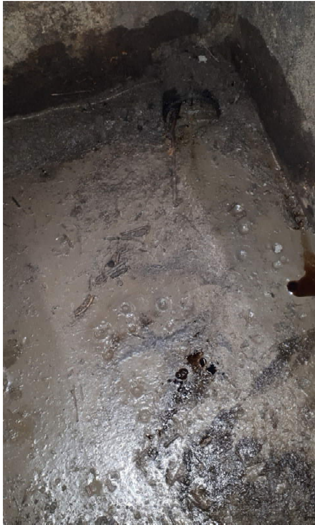
Photograph 7: View of the floor pit with drainage pipe and residual oil in the second (east) garage bay.
