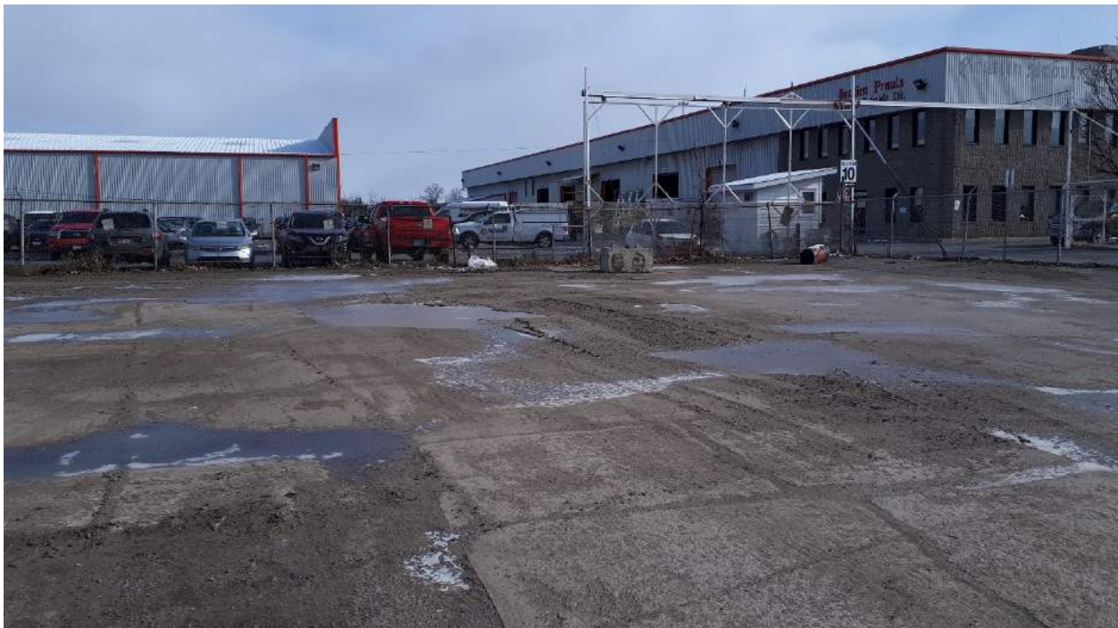
Photograph 2: View of the paved area to the south of the subject building; the former AST slab is visible at bottom-right.
