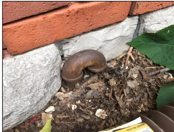
Photo 5: The Phase One Property (28 Pretoria Avenue – historical heating oil AST fill/vent pipe, exterior west wall)
