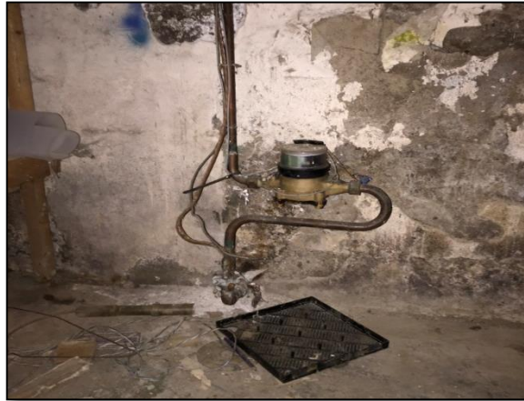
Photo 14: The Phase One Property (30 Pretoria Avenue – general interior view of basement remaining heating oil AST connections)
