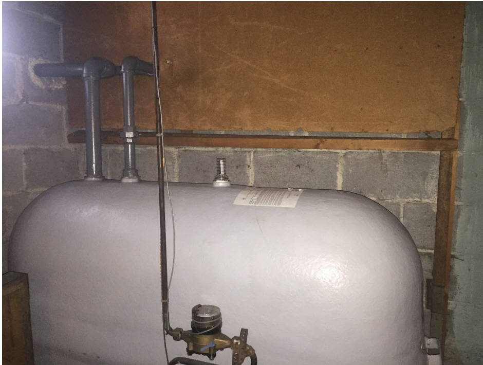
Photo 3; Above ground fibreglass furnace oil tank located in the basement.
