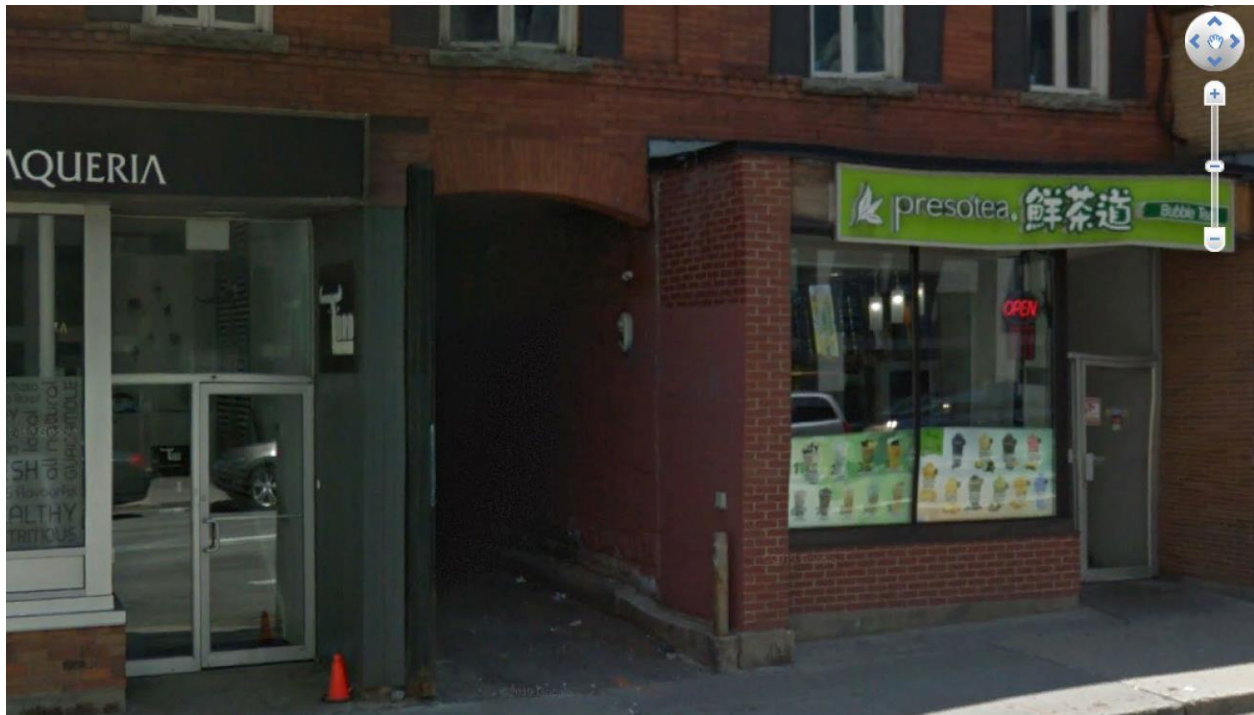
Figure 10: Detail view of the storefront on 208-212 Slater. It would appear that the projecting brick walls, and panel below the storefront window are contemporaneous with a more recent rehabilitation of the storefronts. The same brick detailing is evident on another commercial bay. The original residential configuration consisted of a single window, and door set in the exterior wall aligned with second storey windows. The ground floor exterior walls have been removed, and a beam inserted to support the second floor in order to accommodate the commercial units. The building is classified as a Category 3 heritage resources. Source: Google Earth
