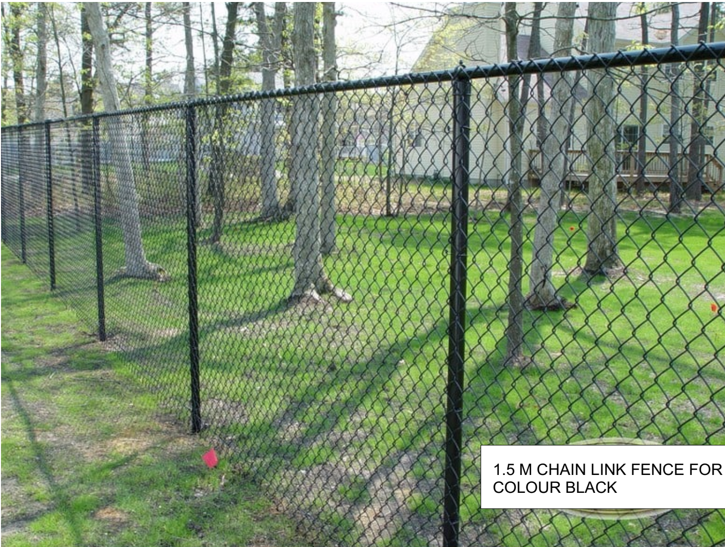
5 CHAIN LINK DOG RUN FENCE N.T.S.
