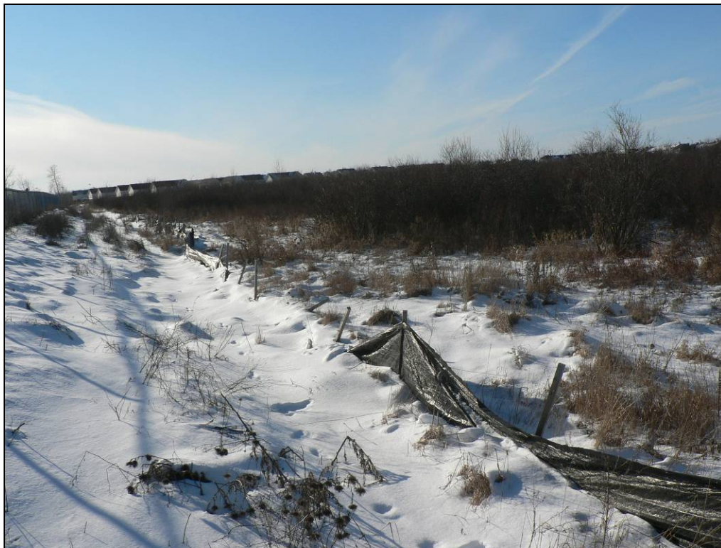
Photo 4: Photo of the silt screen fencing at south east portion of the Site (Parcel B) adjacent to the neighbouring French public school/daycare center. The fencing is inferred to be a remnant of construction activities associated with this facility.
